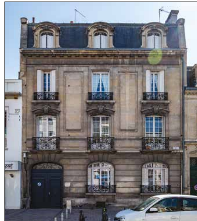
PC 62 – 39, rue Buirette 1920 PC 1732 – 39, rue Buirette 1922
