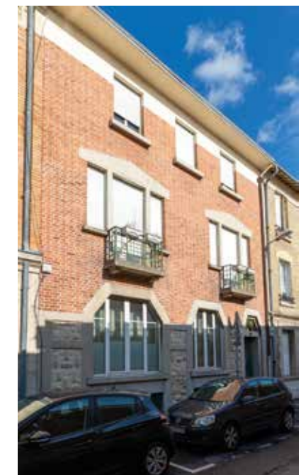
PC 2850 – 11, rue Saint-Pierre-les-Dames 1923
